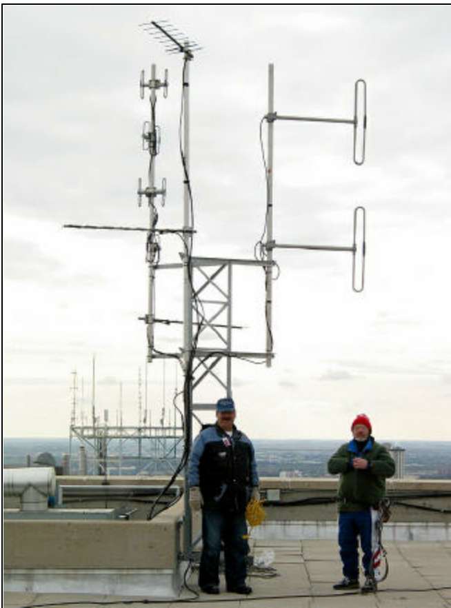
New Tower on top of the Richardson Bldg. VE4GWN & VE4HK helped in the install. Left Mast - Bottom UHF yagi to VE4MAN, Top, 8 bay UHF for VE4VJ. Middle mast - Bottom UHF beam to VE4MIL, Top UHF Beam to VE4GIM. Right Mast - VHF 2 bay for VE4WPG & VE4WRS
